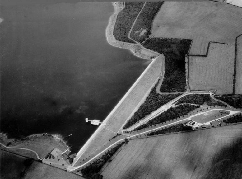
Aerial photographs of Eye Brook reservoir taken on 20th August. 1957. Reservoir level 220.91 feet 0.D. - 6'6" below top water level - holding 1,132 million gallons.
